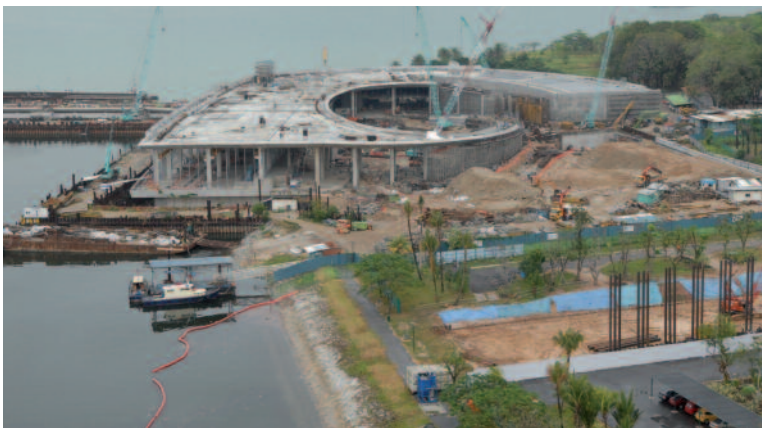
Visitor centre pump station under construction. Credit: PUB Singapore
