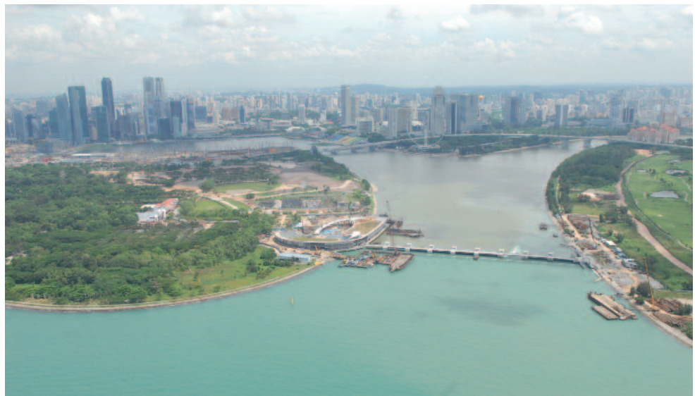
Aerial photograph of the Marina Barrage construction site. Credit: PUB Singapore
